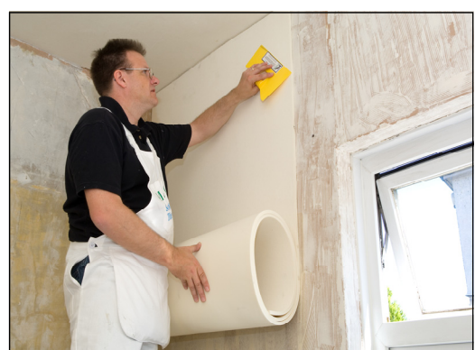
Installation of Sempatap
